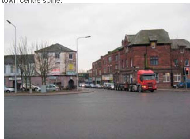
5.19 Conservative Club and former Drill Hall Ashley Way cuts through Victoria Road along the route of the old Central Railway. The pedestrian environment at the crossing is a major severance point between the town centre and West Bank, which contains key attractions in Spike Island, the Catalyst Museum and Victoria Promenade.
