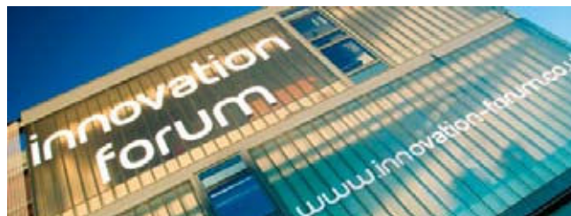
Salford Innovation Forum is a £9m project combining business incubation and community facilities.
