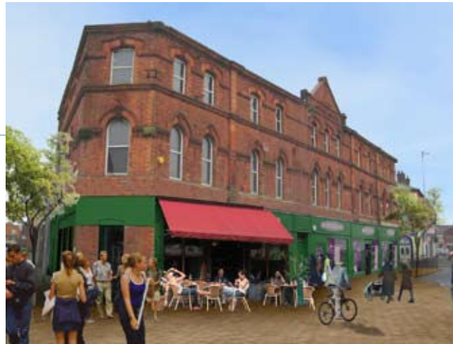
Intervention should aim to activate the ground floors to add life to Victoria Road. Shutters and shop fronts should enhance street
